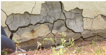
Cracking foundation
